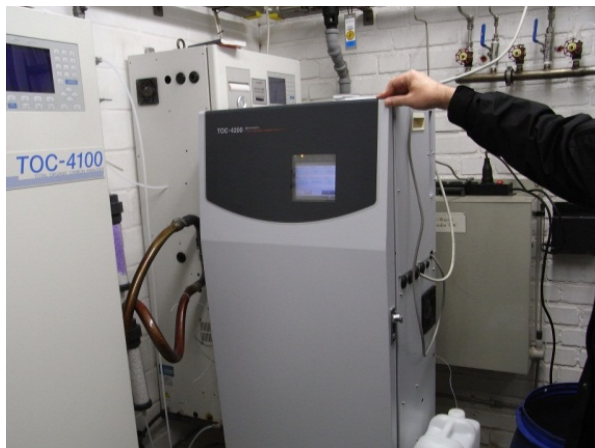
Fig. TOC-4200 on site
